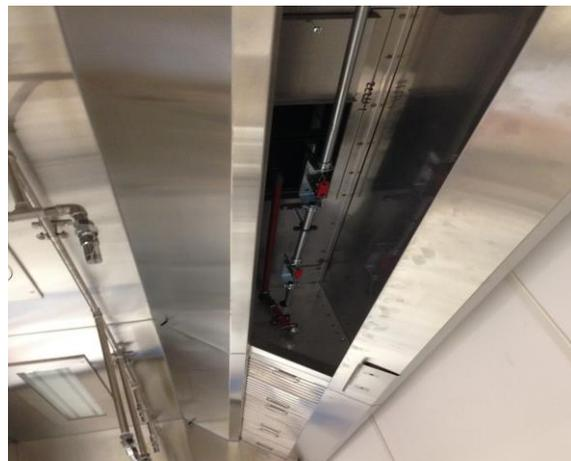
Heat sensitive fusible link valve located in extract plenum which activates suppression system **3 of 9**
